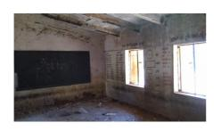
A badly damaged classroom as a result of a leaky roof. Most classrooms in a similar, barely useable condition.
