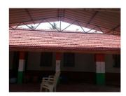
Tile roof repaired and broken tiles replaced all around
